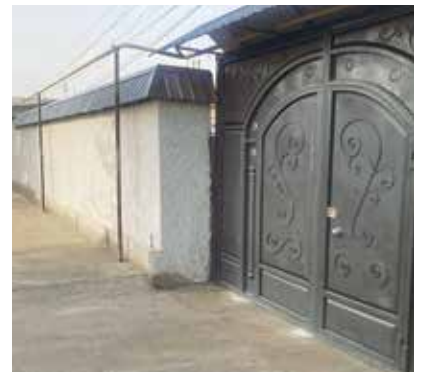
Barnabas-funded repairs restored the church's flood-damaged perimeter wall
